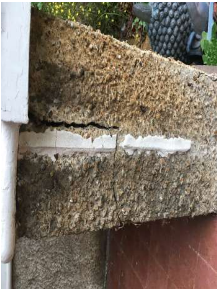
Photo 11 - Porch photo No. 2
