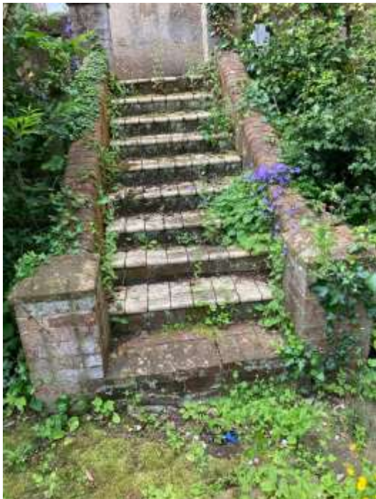
Photo 3 - Overgrown paths & stairways - dangerously uneven
