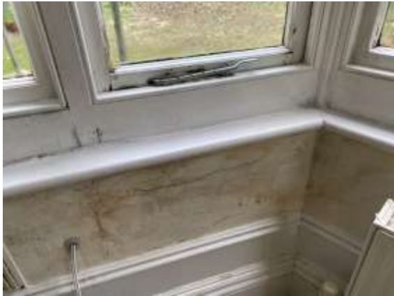
Photo 2 - A ground floor flat
